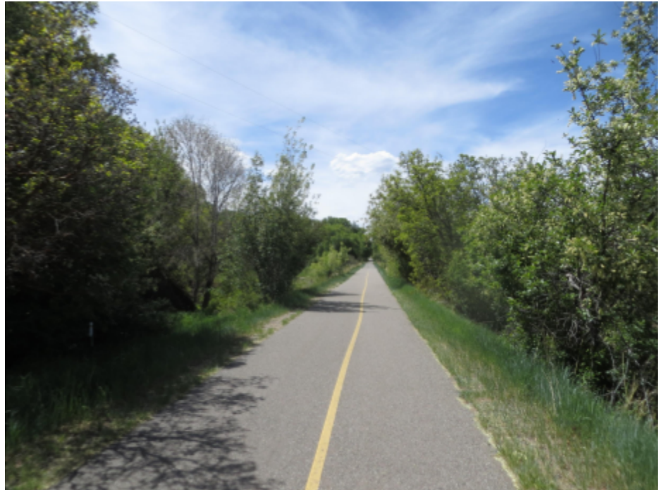
The Rio Grande Trail in Eagle County heading north towards the Garfield County line. Photo: Eagle County
