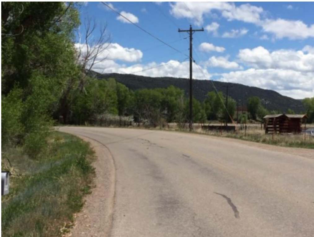
Valley Road near the USFS Fishing Access entry, to the right. Photo: Eagle County
