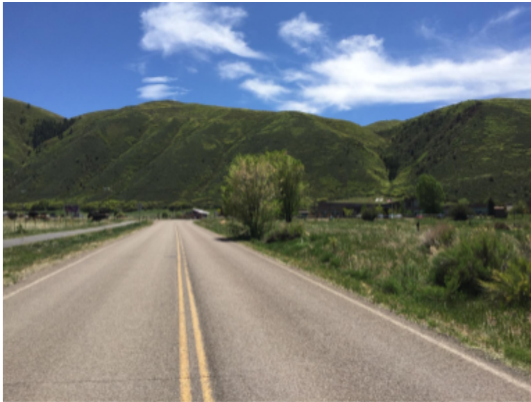
Southside Drive, looking towards Basalt High School. Photo: Eagle County
