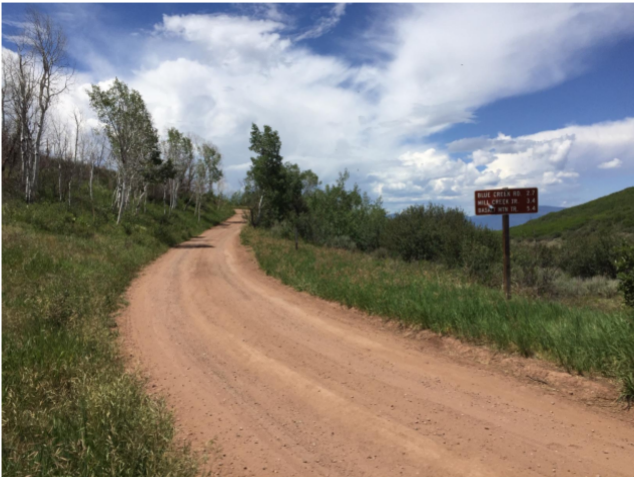
Basalt Mountain Road access to singletrack trails. Photo: Eagle County
