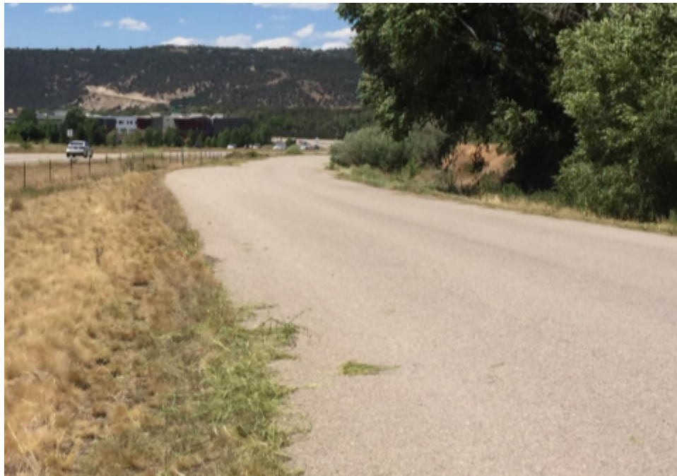
SH 82 North Frontage Road right-of-way is a potential connector to link Two Rivers Road to the Tree Farm PUD. Photo: Eagle County
