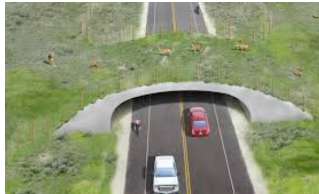
Group Looks To Protect Drivers & Wildlife On Highway 9 – Silverthorn, CO
