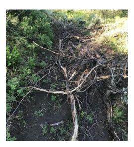
Time was spent on old erosion wash areas by filling steep gullies with earth & brush, while creating water run off channels away from the new switchback trail.
