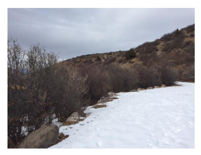
Left side of the parking area needs to be enlarged. Pulling material from the uphill side of this area can be used as fill to widen the left downhill portion. The large rocks can be pulled from the left side and used to support the right, uphill side of this parking area to prevent erosion, and secure the right, side bank.
