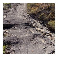
Water damage in places on the shale hill of Upper North Mesa Trail also needs attention. Drainage work from above the hill and water bars can be put in place to prevent wash out damage.
